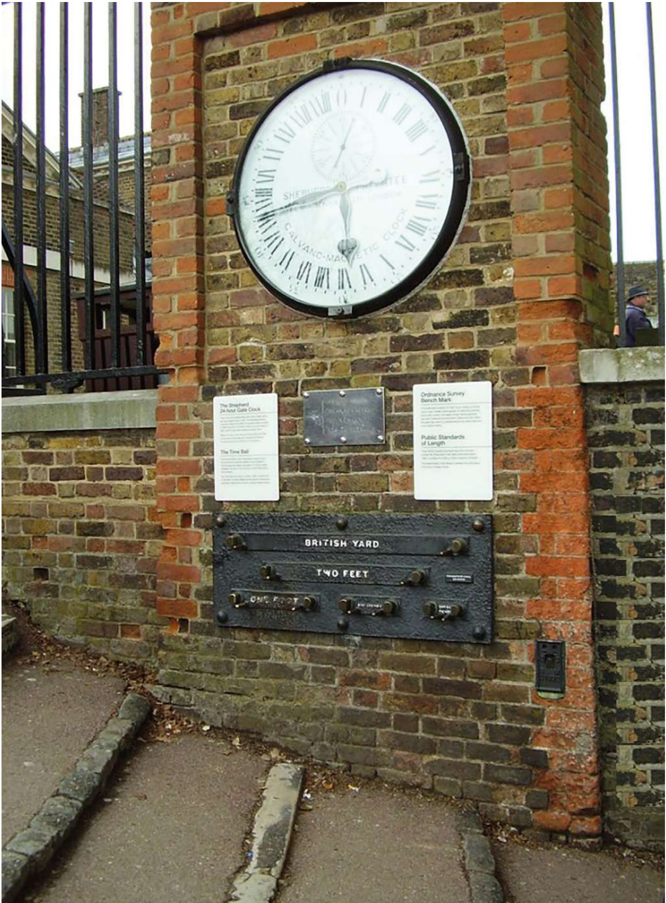
The Shepherd Gate Clock is mounted on the wall outside the gate of the Royal Greenwich Observatory in Greenwich, Greater London. The clock, a prime example of electric clock, was a slave mechanism controlled by electric impulses transmitted by a main clock inside the main building. The master and slave watch network was built and installed by Charles Shepherd in 1852. The clock near the gate was probably the first to show the average Greenwich time to the public and it is unusual to use the 24-hour analogue dial.
